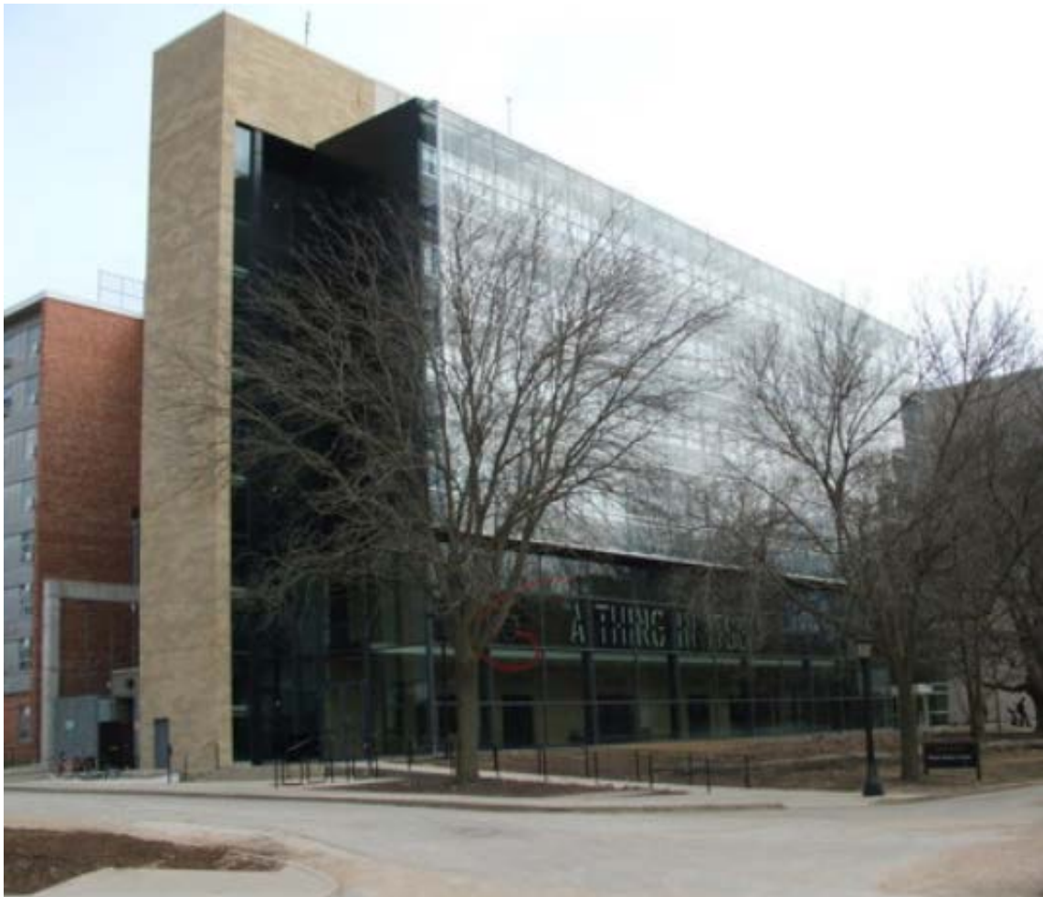
Figure 2.3 Envelope - Northwest view
